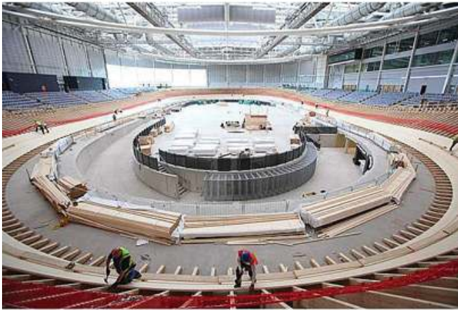
Figure 29: Specialized velodrome installation companies build and install the track.
