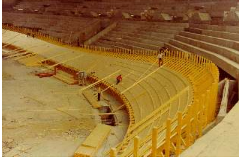
Figure 28: Velodrome track construction after completion of the building envelope.
